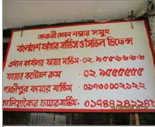
Photo of fire safety equipment Emergency telephone number posted.JPG
